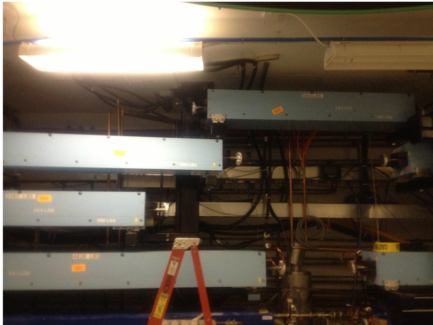
West Arc Stack 16 Magnets in place!
