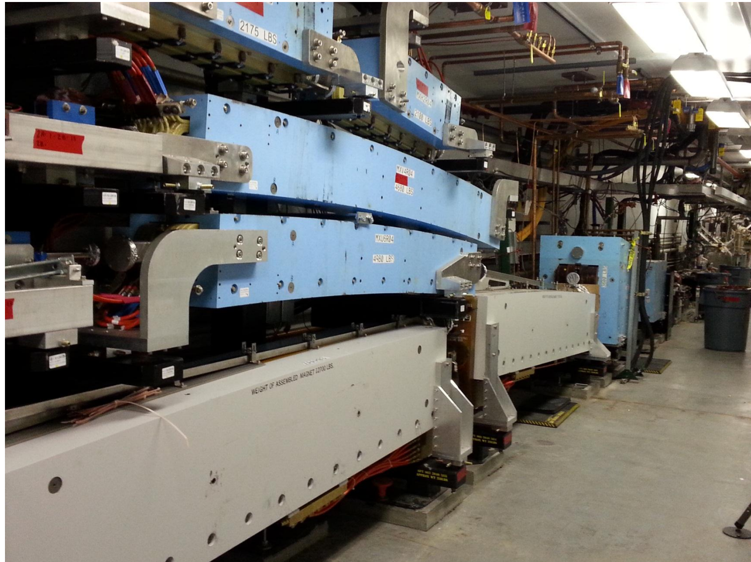
2R + ZA's in place
