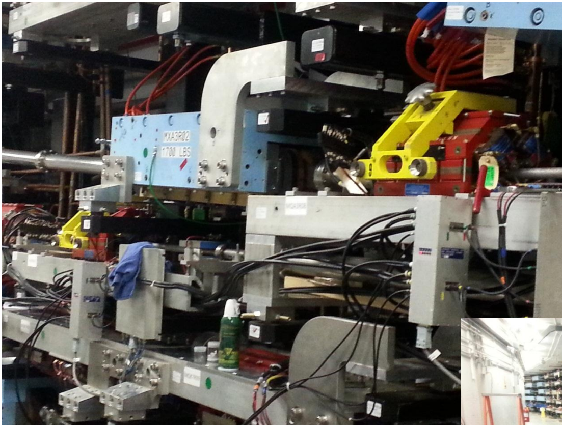
ARC 1 and ARC 3 undergoing alignment
