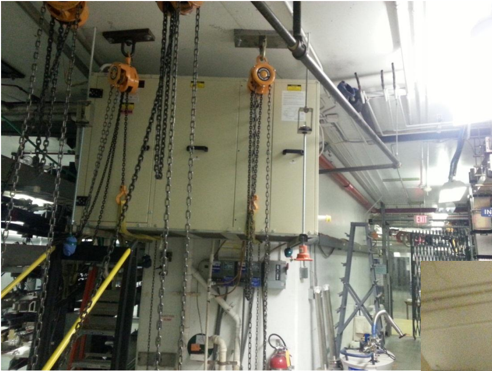
Injector dehumidifier under installation & installed
