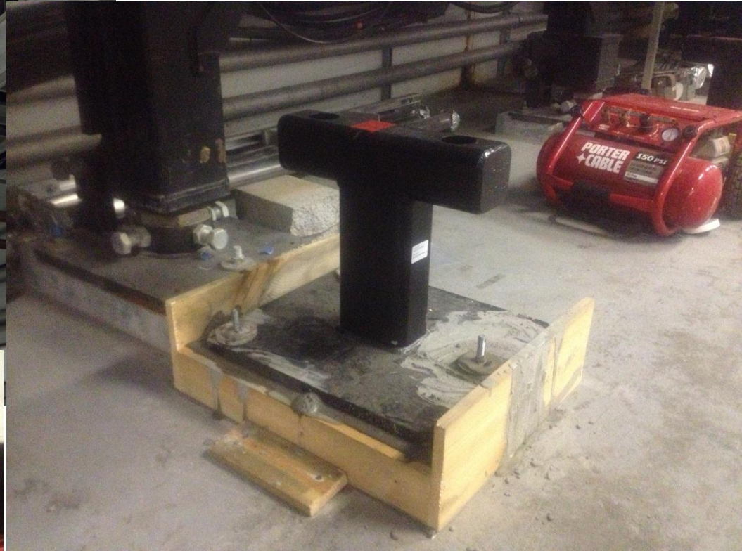
Pedestals 2E+ grouted
