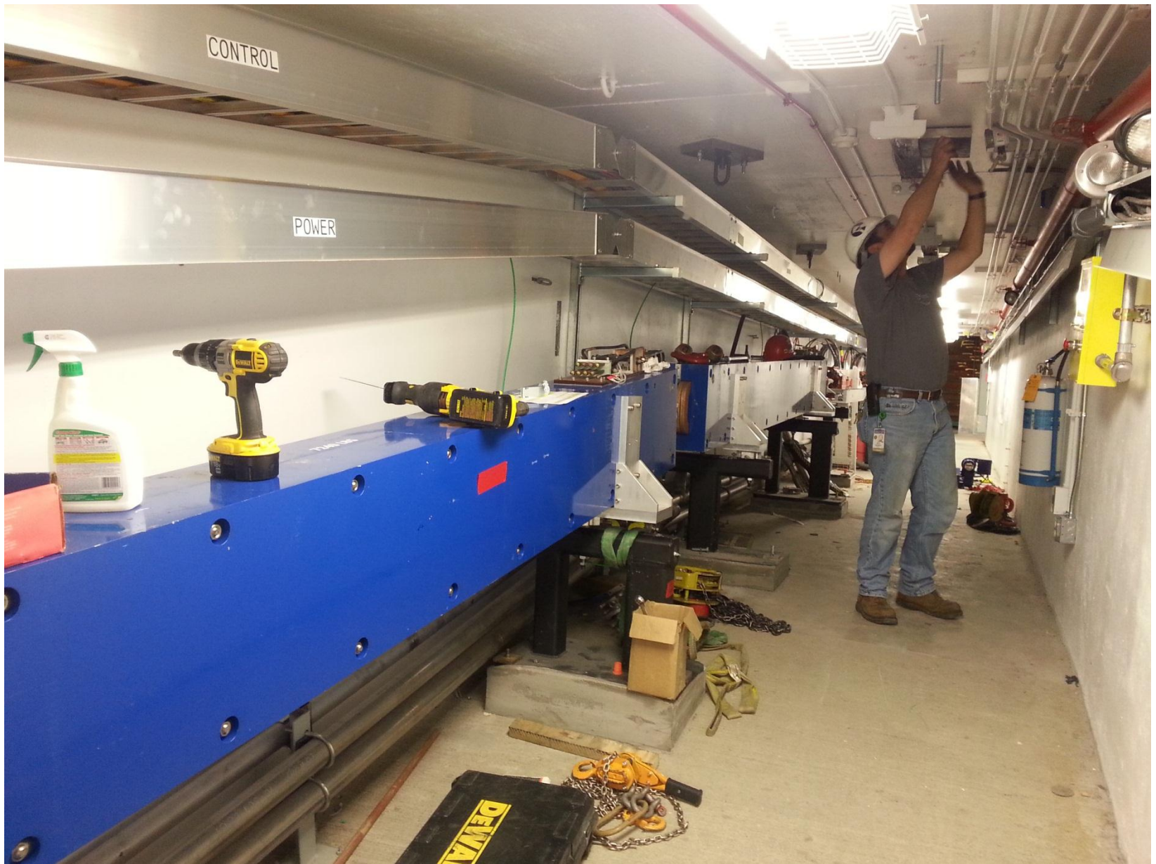
XD line 4 meter dipole installation
